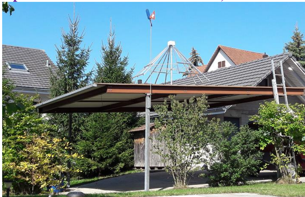
Fig. 5: LWA from Peter H. in Muhen has been moved to the roof of the garage.
