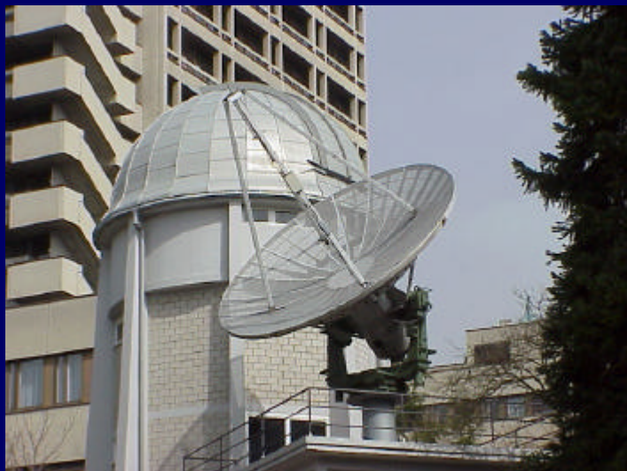
5m antenna Zürich 1 ... 8.6 GHz (system tests only)
