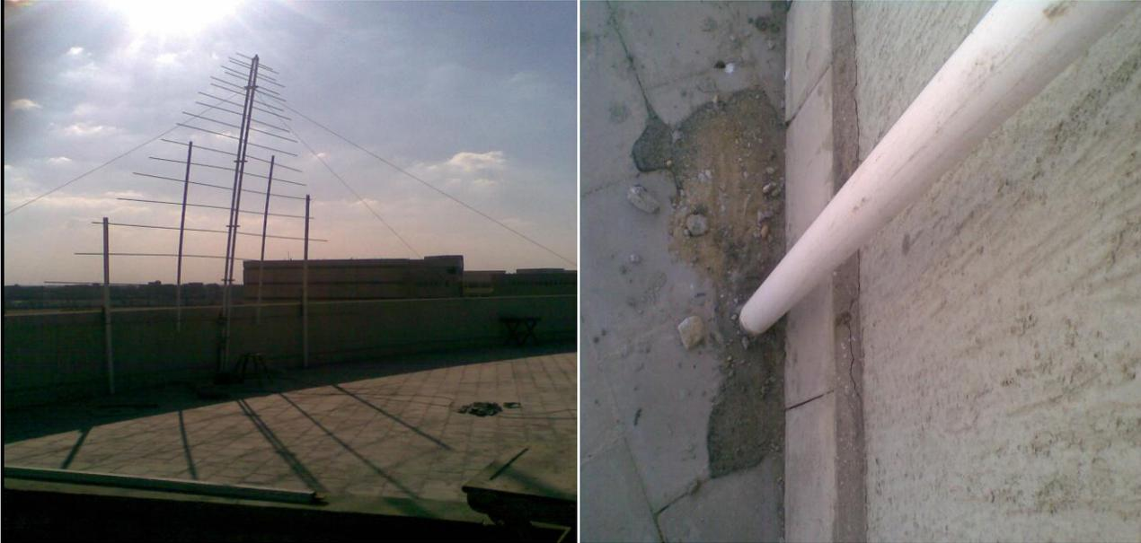
*We fixed the plastic tubes & the al. bars in the roof, as to be fixed, also we applied 3-roped from different positions in order to fix it from everywhere so it will resist the wind*
