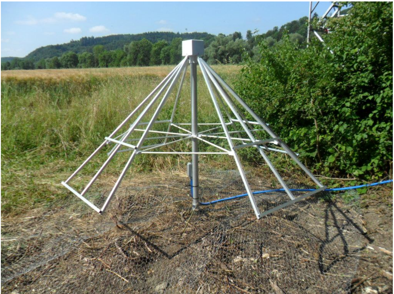
Figure 1 ~ An LWA antenna installed at the observatory site in Bleien, Switzerland. Chicken wire mesh on the ground is meant as ground reflector. The blue plastic tube contains two coaxial cables (one per linear polarization) going to the observatory.
